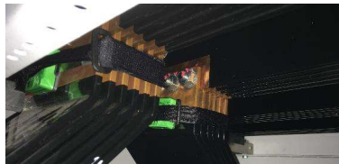
Withdrawable Circuit-breaker (Upper, Lower arm)
